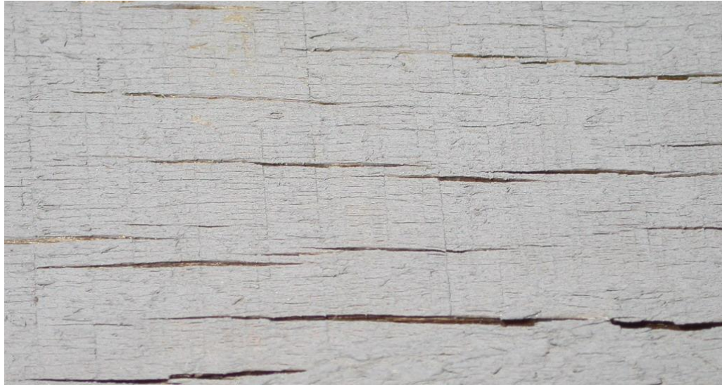
Figure 24 Checking on wood product with a weathered penetrating stain coating
