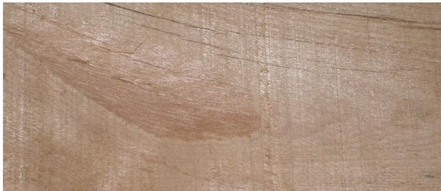
Figure 15 Shakes occurred alone with wood grain of a board
