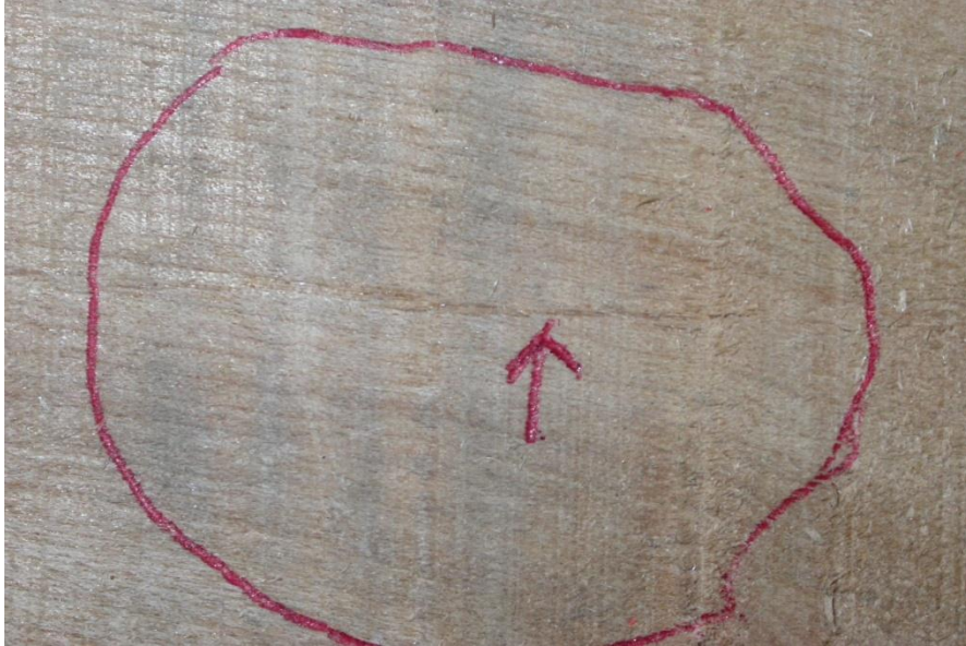
Figure 6 A micro-check occurred on a rough surface of a board
